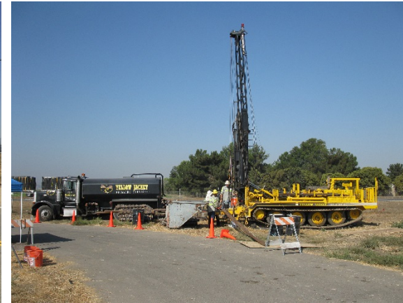
Track-mounted hollow-stem auger drill rig installing monitoring wells on southern boundary of the Airport Property .
