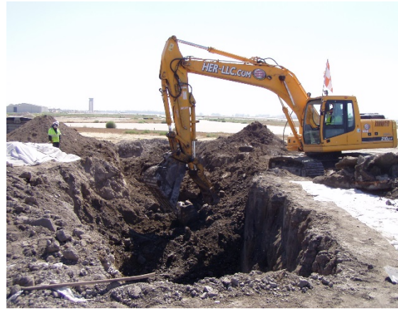
Removal of buried drums, debris, and impacted soil discovered during trenching for installation of a storm drain pipeline for a new Southern California Edison facility at the Airport .
