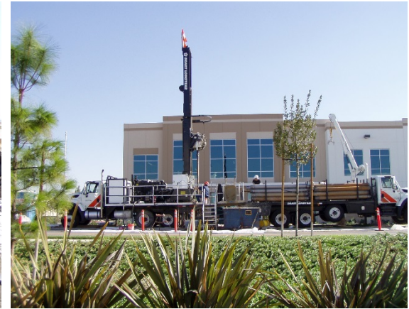
Sonic rotary drilling rig used to install off- Site monitoring wells southwest of the Airport to delineate the off- Site trichloroethene (TCE) plume.
