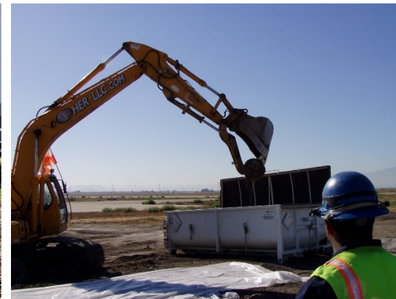
Large excavator used to remove buried drums discovered during trenching for installation of a storm drain pipeline for a Southern California Edison facility at the Airport .
