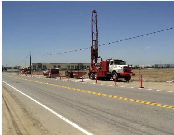
Hollow-stem auger drill rig used to install off- Site monitoring wells south of the Airport .
